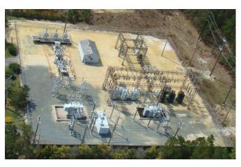
Figure 5 - Distribution Substation
